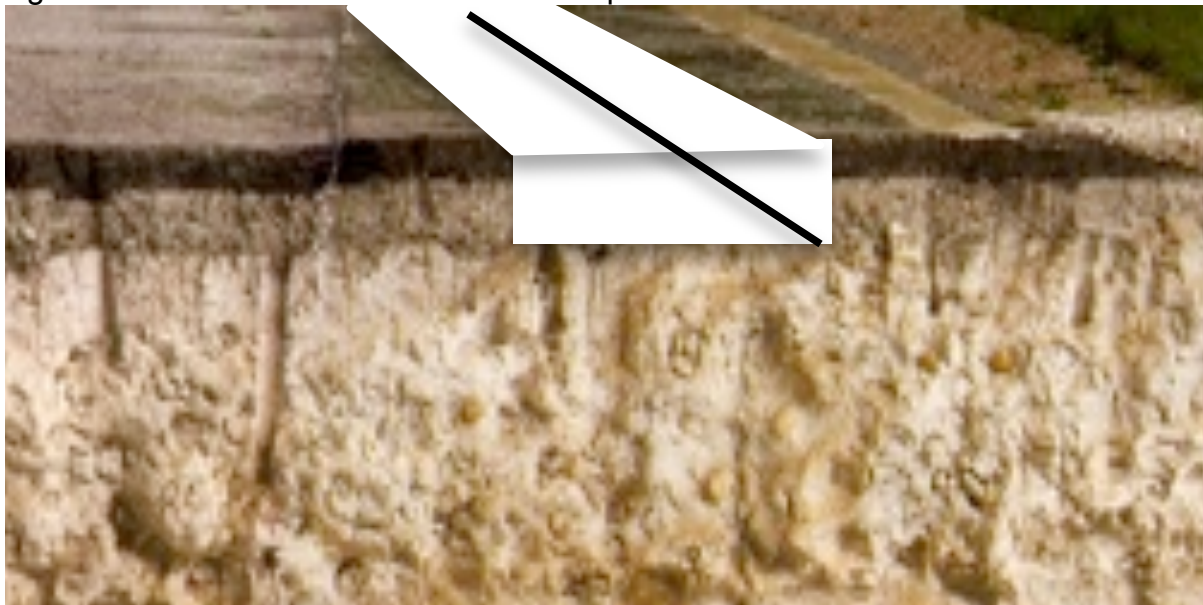
Fig. 2 Rotherham bus station schematic: apron excavated for LR55 beams
