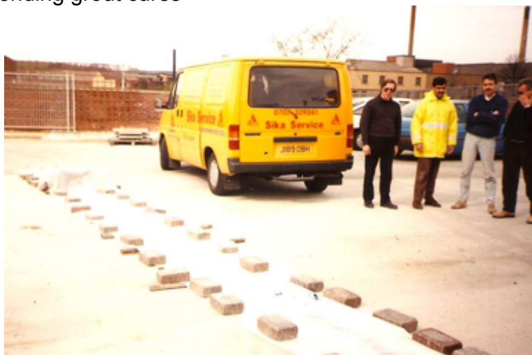
Fig. 9 LR55 bonding grout cures
