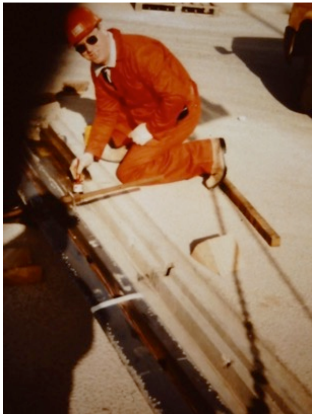
Fig. 4 Priming the rail and beams
