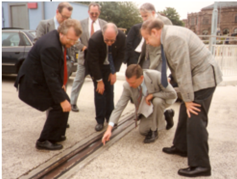
Fig. 13 6 month inspection team
