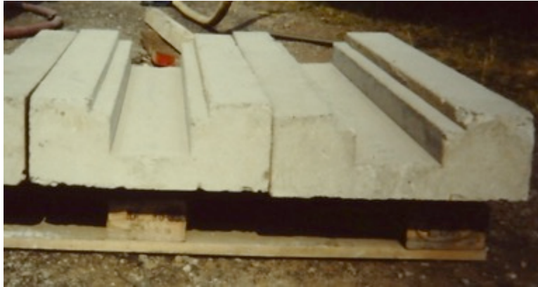
Fig. 3 LR55 Pre-cast 40N concrete Foundation Beams delivered to site
