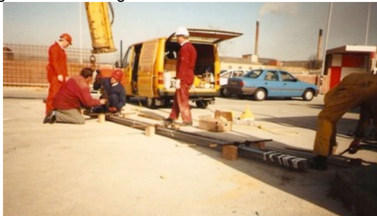
Fig. 7 Adjusting LR55 rail for alignment
