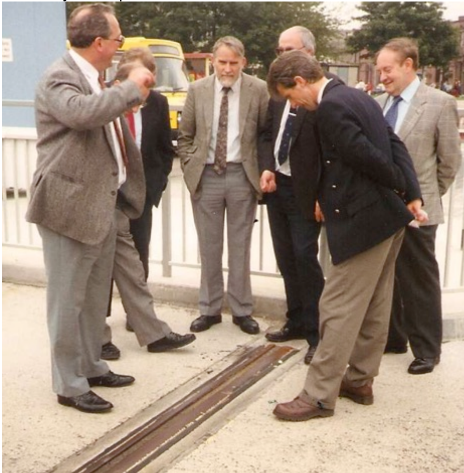
Fig.16 Two year inspection
