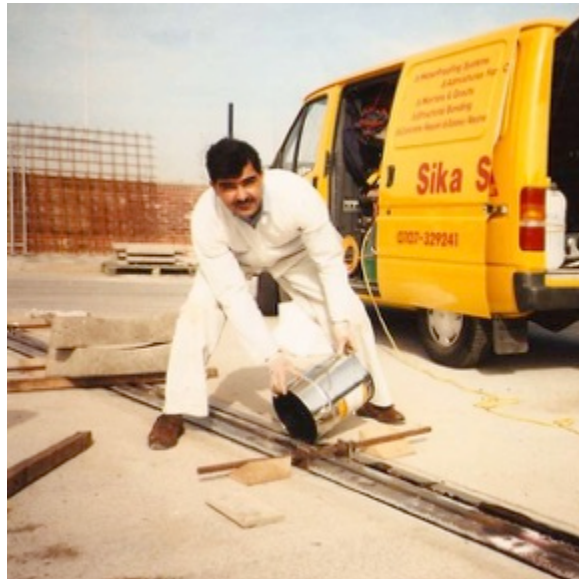
Fig. 8 Bonding LR55 rail to foundation beams
