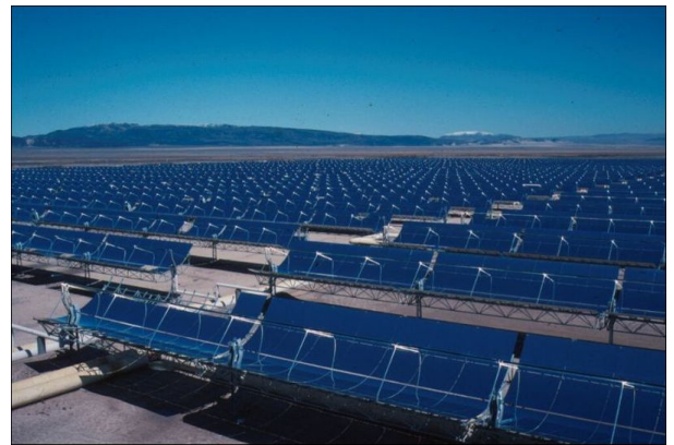
Parabolic trough collector field for the solar thermal power plants in Kramer Junction, California
